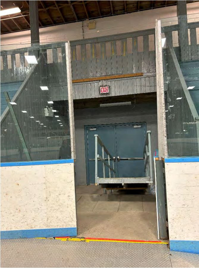
Sample Exit Sign to be replaced
