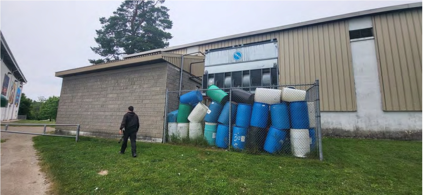
Ice Plant Condenser
