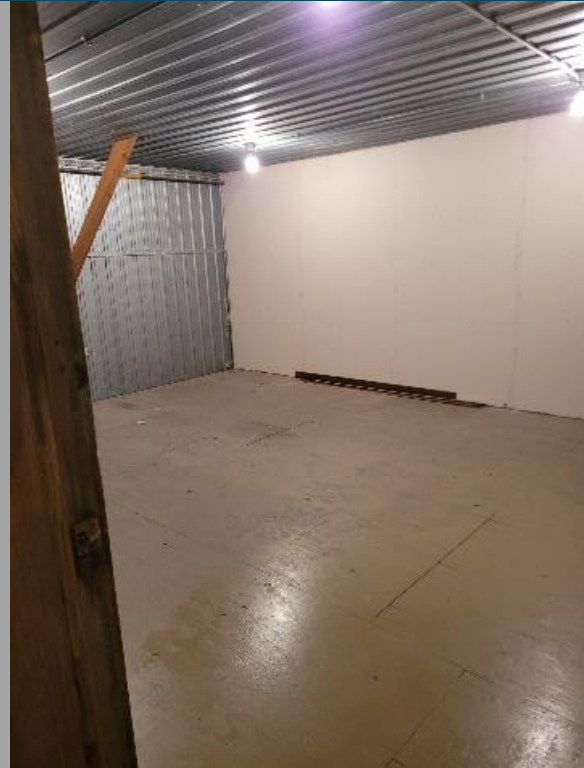
Second Floor Archive/Storage Room
