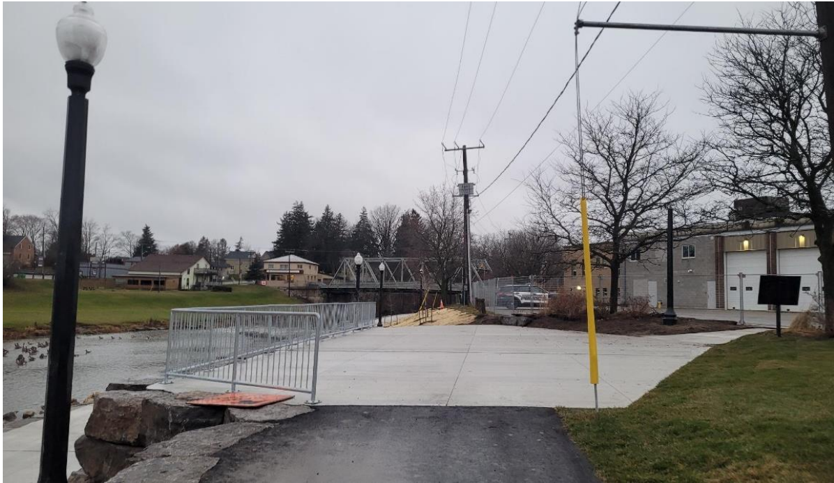
Nith River Trial Upper Gathering Space Post Construction
