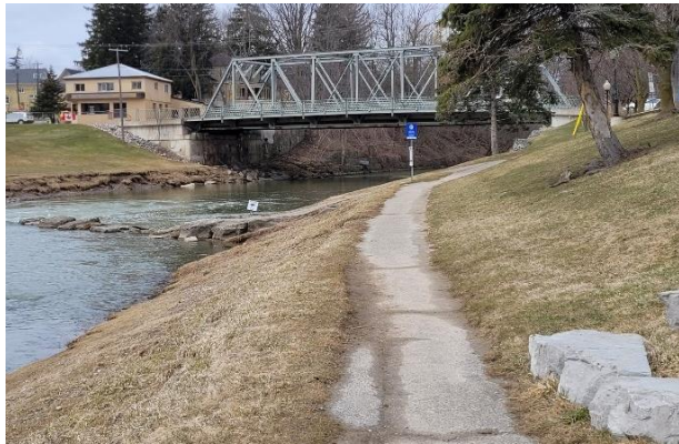
Nith River Promenade North Headwall & Portage Pre-Construction
