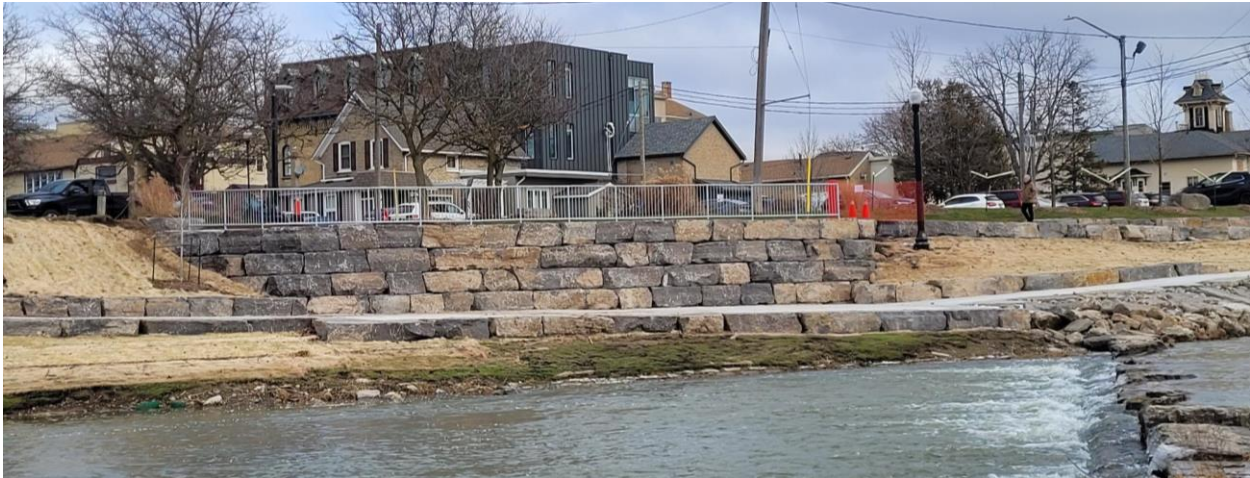
Nith River Promenade Upper & Lower Gathering Spaces Post-Construction
