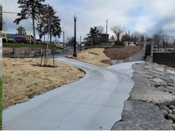
Nith River Promenade Accessible Ramp Connection Post-Construction
