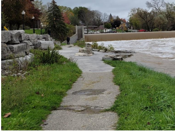
Nith River Promenade Accessible Ramp Connection Pre-Construction
