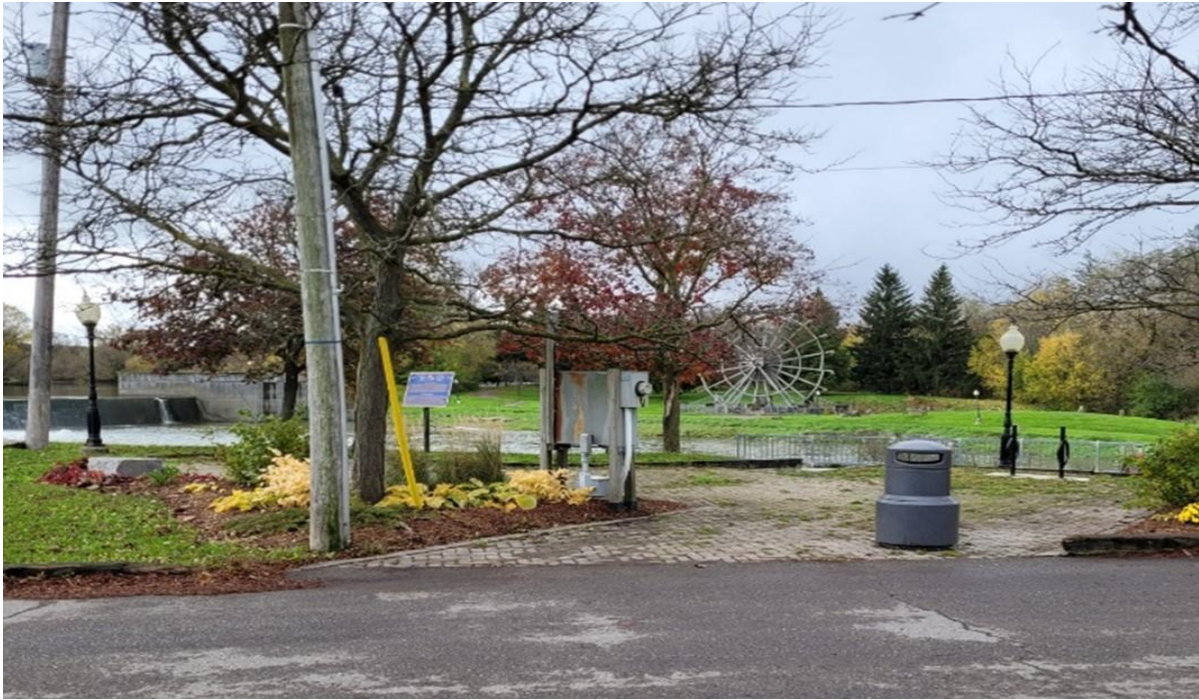
Nith River Trail Entrance to Upper Gathering Space from Huron Road Pre-Construction
