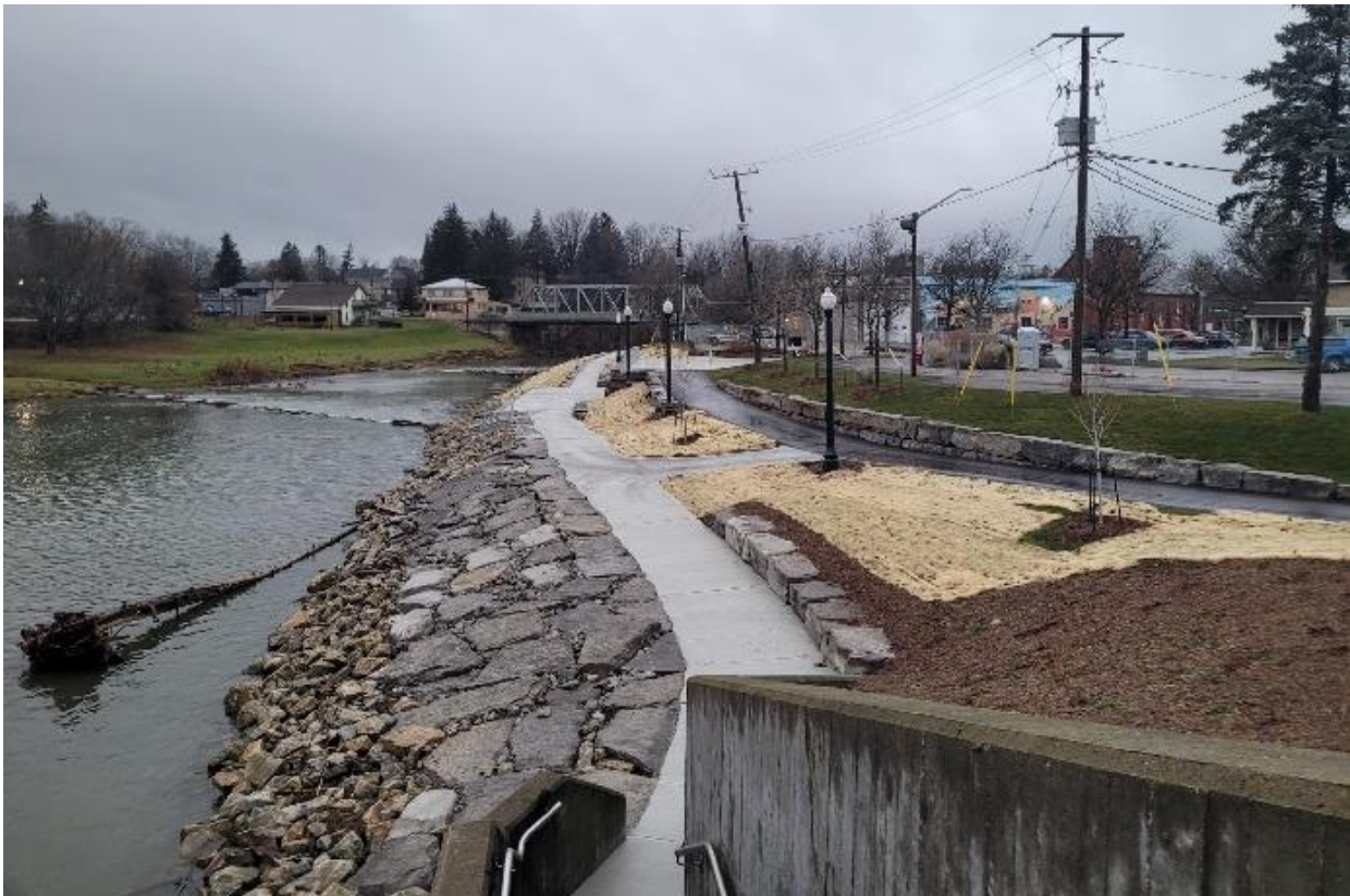
Nith River Promenade & Trail (South) Post Construction
