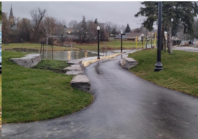
Nith River Trail (South) Post-Construction
