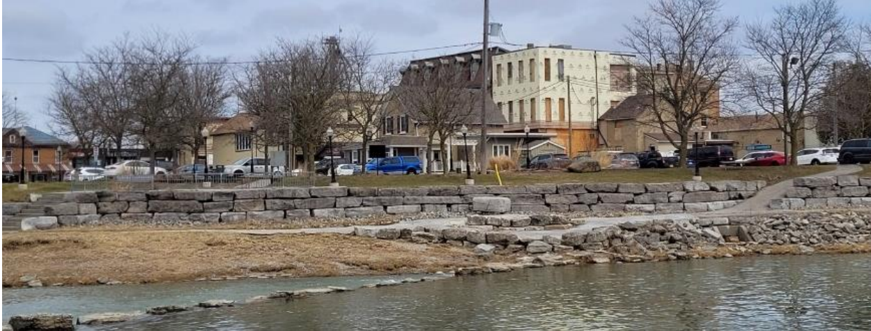
Nith River Promenade Upper Gathering Space Pre-Construction
