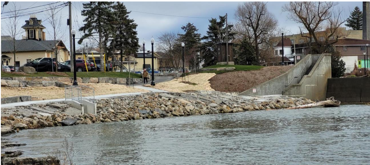
Nith River Promenade (South) Post-Construction
