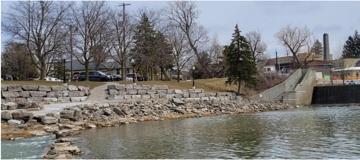
Nith River Promenade (South) Pre-Construction
