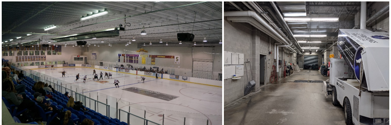
Wilmot Recreation Complex Event Rink & Ice Resurfacer Corridor
