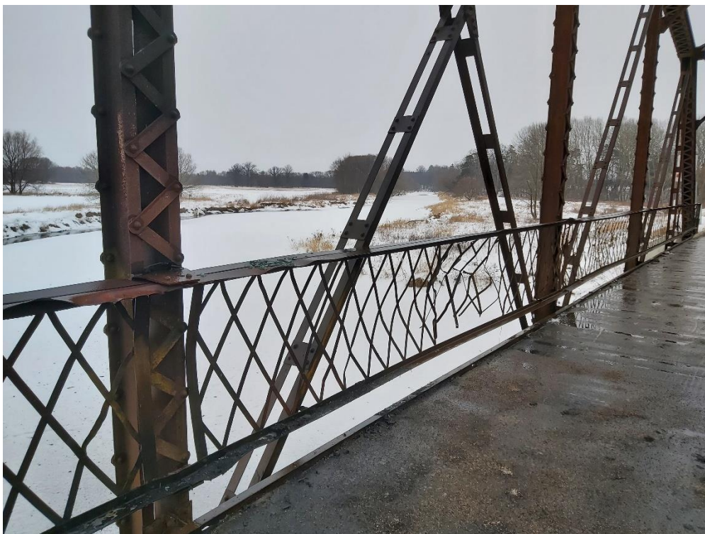
North Side, fourth bay from east end – heavy damage to railing panels. Also note blackened area at deck and structural members.
