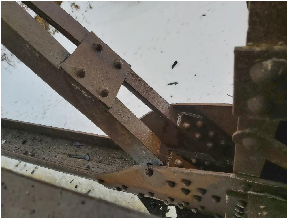
South side, third bay from east end – damage at diagonal structural member. Interior angle is completely broken above connection plate location.
