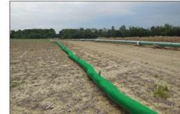
Filtrex SiltSoxx ORIGINAL used as Perimeter Control.
