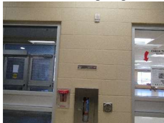
39 - Fire pull and extinguisher and visual alarm placement
