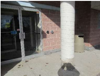
8 - Entrance, no contrast on support beam
