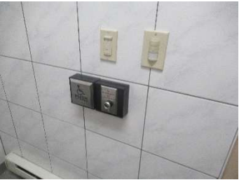
87 - Wilmot Community Centre, Universal Washroom, automatic controls and lock
