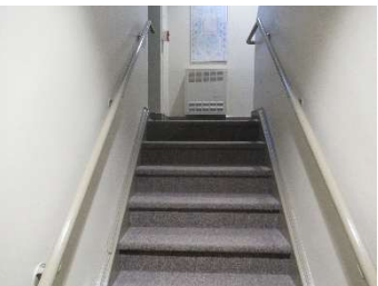
24 - Lower Level - stairwell - low contrast at railings
