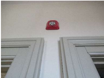
8 - Main Floor - Universal Washroom, visual alarm placement
