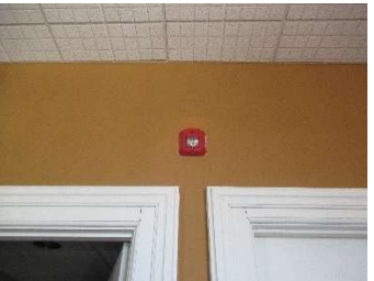
20 - 2nd Floor - Universal Washroom, visual alarm placement
