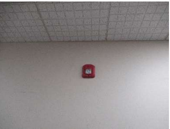
48 - 2nd Floor, Planning and Building, visual alarm
